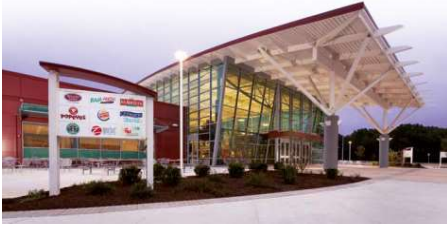
Service areas, professional kitchens and restaurants Servis alanları, profesyonel mutfaklar ve restoranlar
